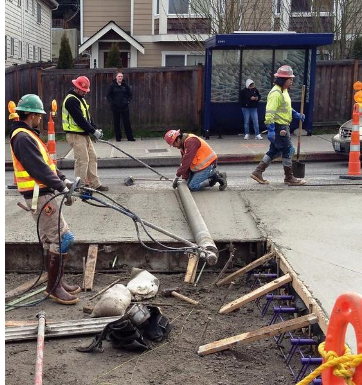
Paving on Delridge Way SW
